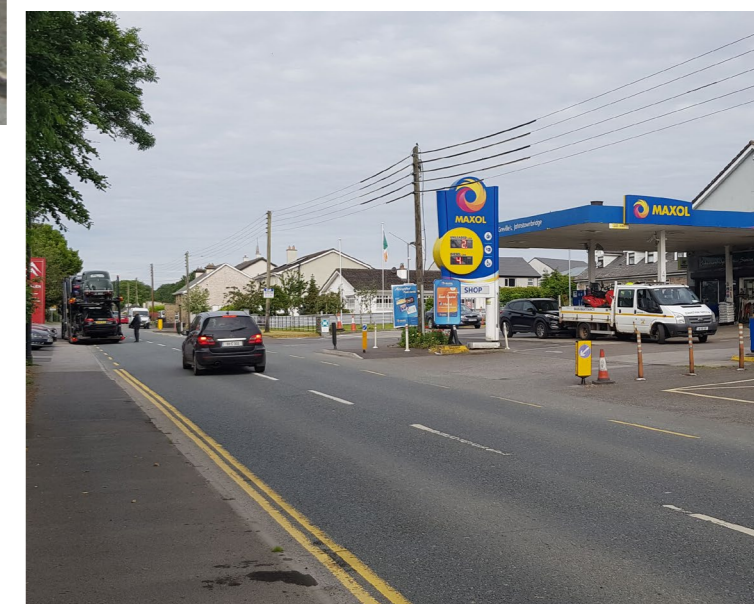
Right: Carriageway at Service station Lack of pedestrian facilities is evident in this area and will be considered in relation to improved movement.
