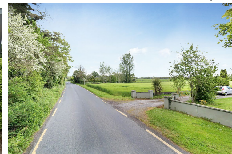
Below: Road to Johnstownbridge GAA There is a lack of pedestrian facilities connecting the village core to the GAA grounds.
