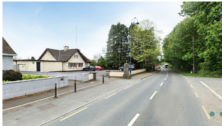
Left: Existing road junction at Johnstownbridge Health Centre.
